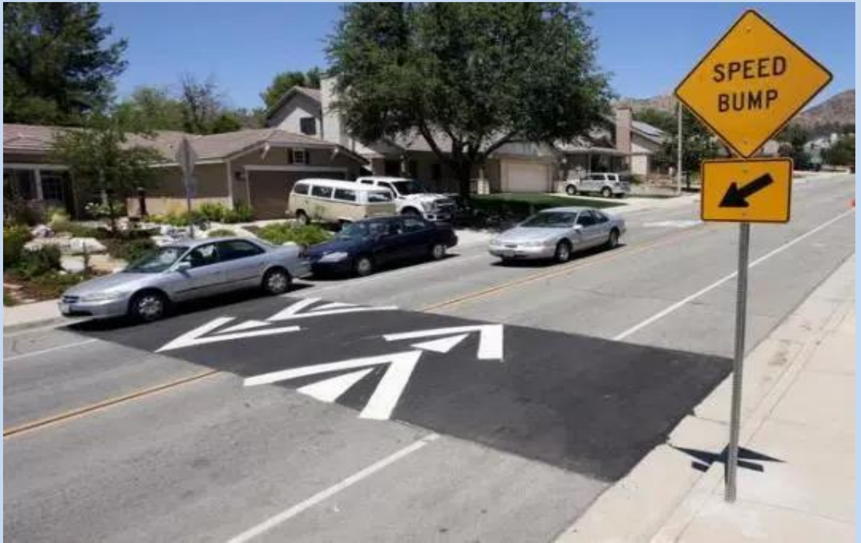
Typical edged to edge installation
