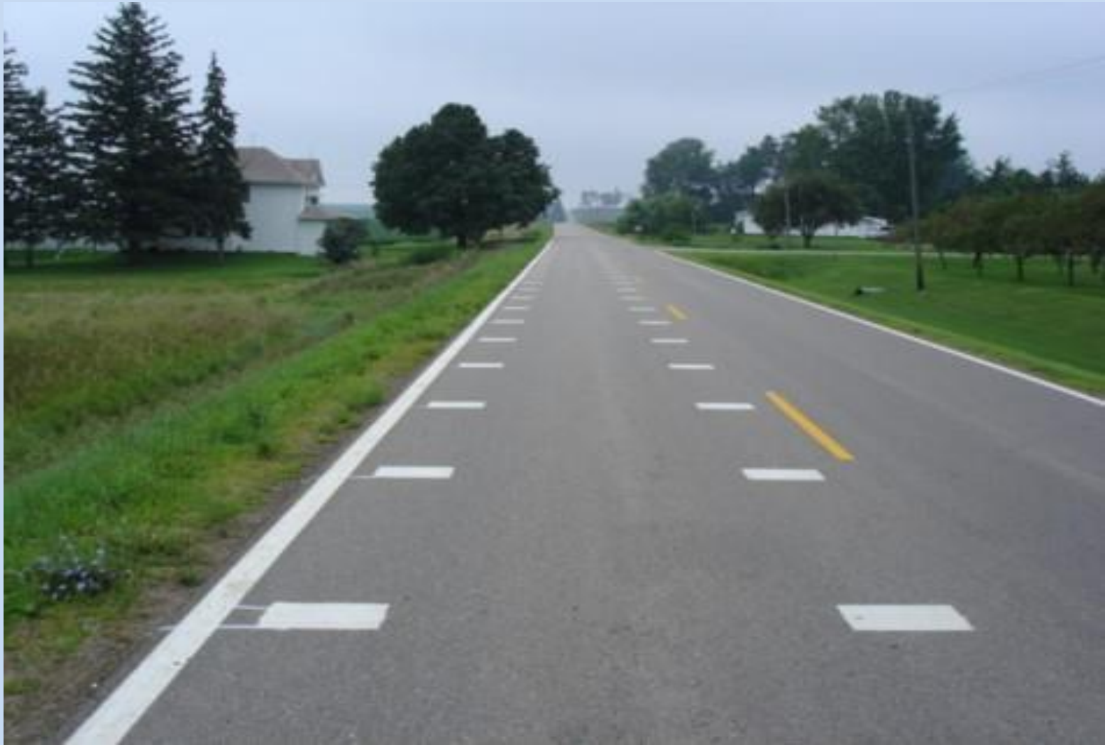
Transverse Lane Markings
