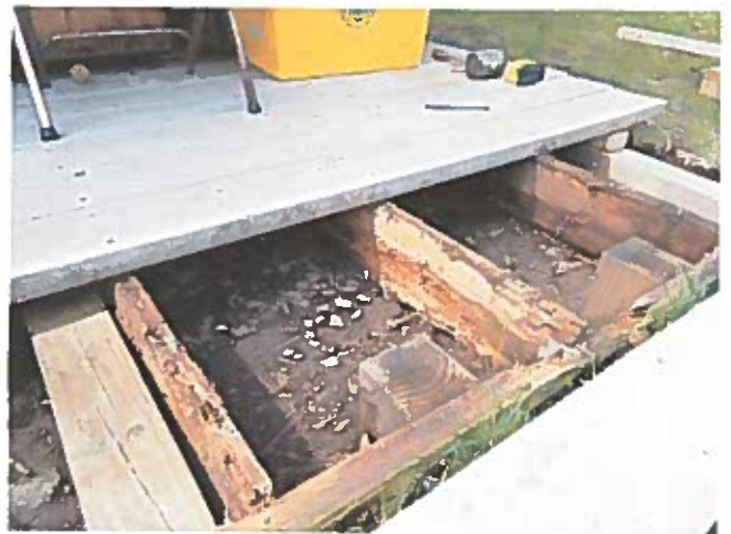
The rotting porch replaced as an Eagle Scout project.
