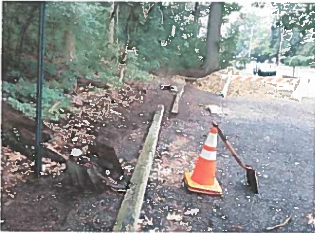
Creating a trail and fixing up the parking lot.
