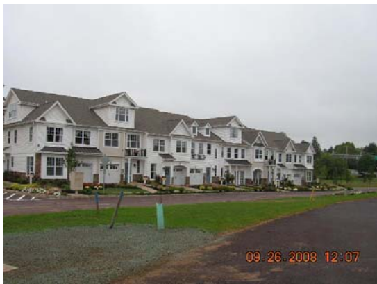
Each home in the new Wyngate development is equipped with a residential sprinkler system
